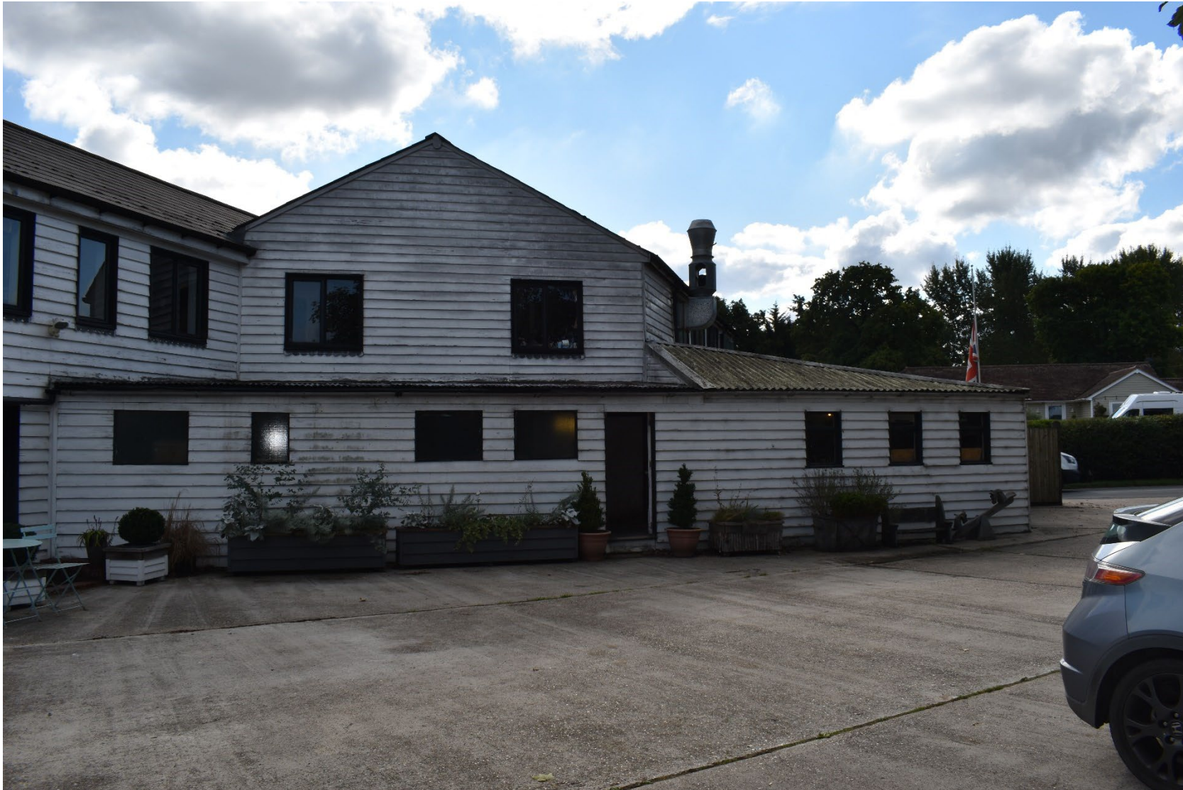
Plate 8: Rear of the building (facing SE)
