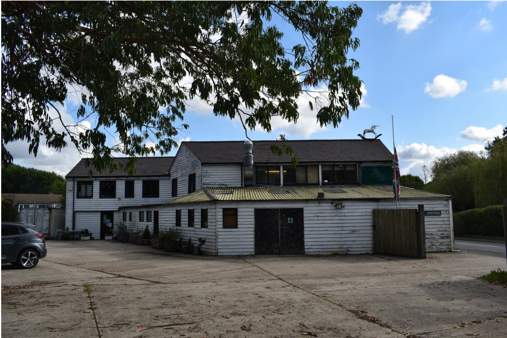
Plate 7: View across the yard (facing ENE).
